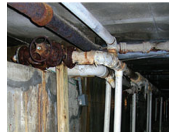
Pool is beyond reasonable repair
